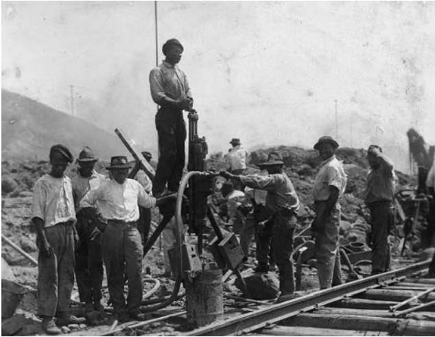
Railway workers with pneumatic drill. Undated photograph.
