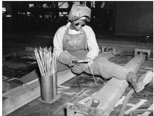
African-American trainee welder Josie Lucille Owens working on the construction of the Liberty ship SS George Washington Carver at Kaiser shipyards in Richmond, California. (1943)
